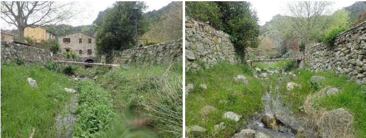
Figure 51 : Passerelle du parking amont du village
