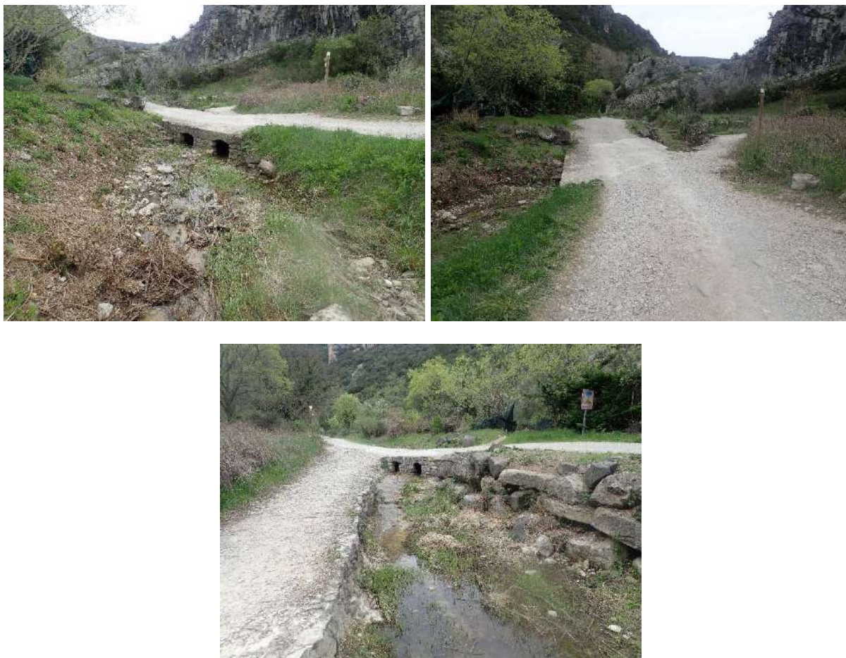
Figure 48 : Ouvrage double buses
